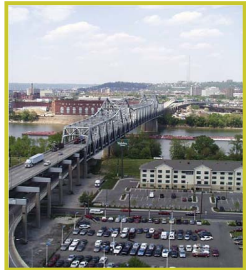
Brent Spence Bridge
