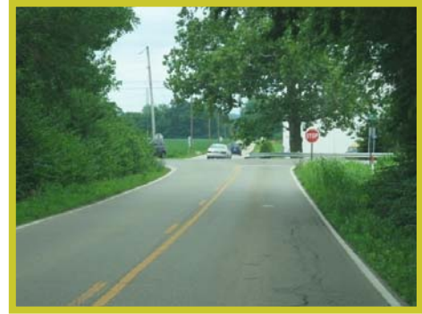
Union Road Improvements
