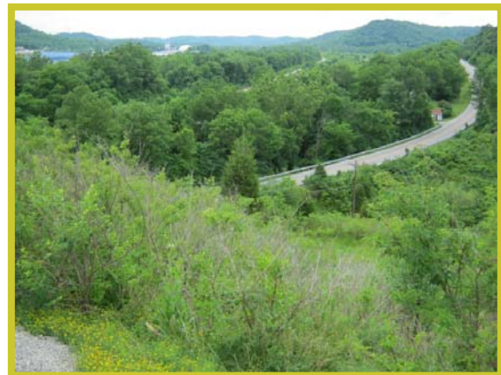
Truck Access South of I-275
