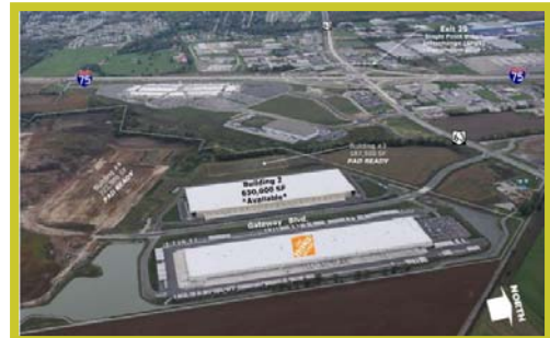
Gateway Boulevard Extension
