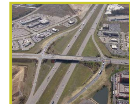
I-75/Union Centre Boulevard Interchange
