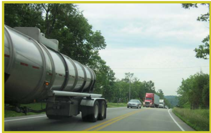
SR 1 Northbound Climbing Lane
