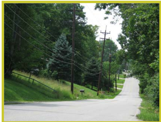
Grand Avenue Improvement, Taylor Mill
